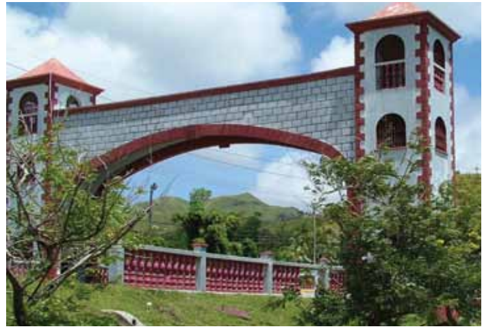
Old Spanish Bridge in Umatac, Guam. Courtesy of the Office of U.S. Representative Madeleine Z. Bordallo.
