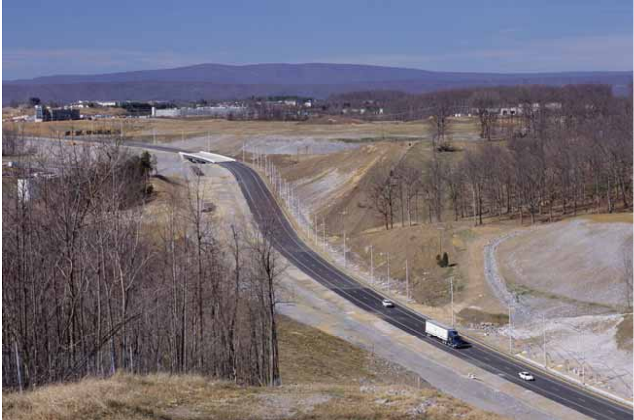
Figure 7. Photo. Smart Road.
