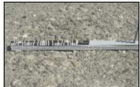
FIGURE 42 Distress Type ACP 13—Loss of Coarse Aggregate
