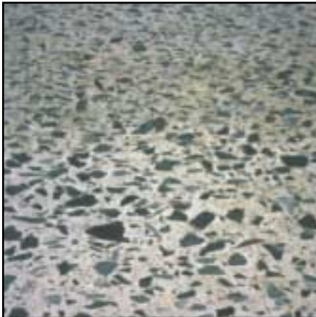
FIGURE 72 Distress Type JCP 9—Polished Aggregate
