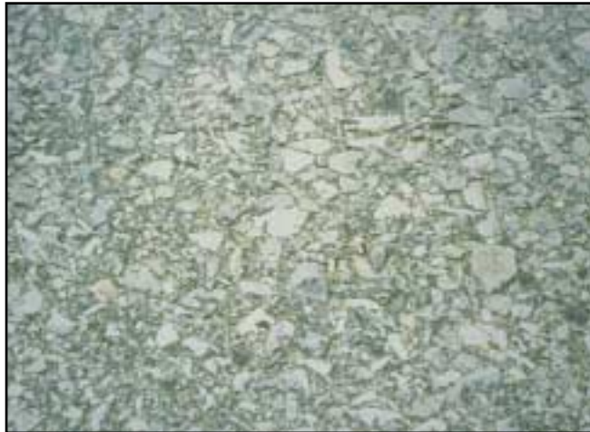
FIGURE 39 Distress Type ACP 12—Polished Aggregate
