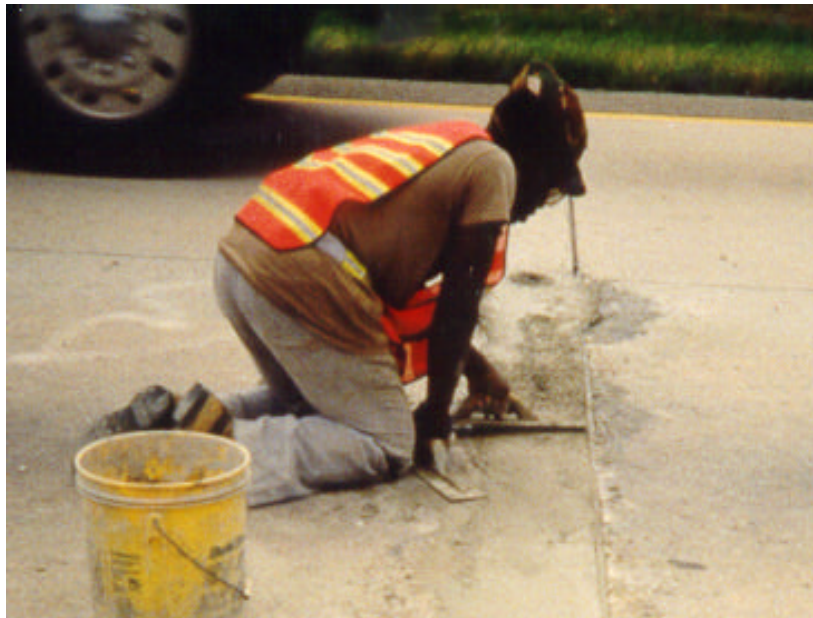
Figure 26. Finishing the patch.
