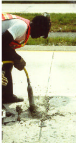
Figure 24. Using an internal vibrator.
