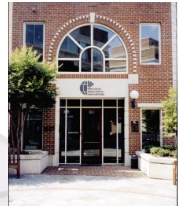
Helicopter Association International (HAI) Headquarters
