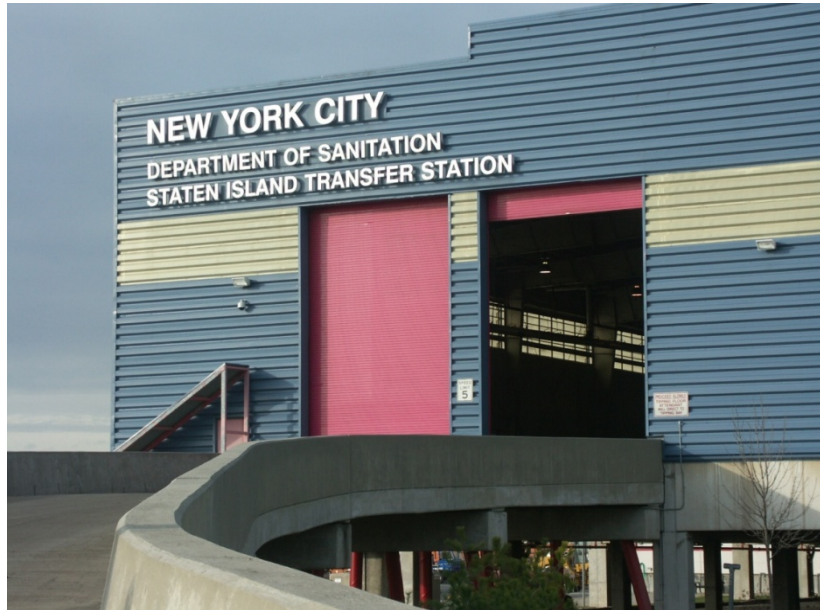
Figure 3-8. Standardized bird surveys were conducted at the Staten Island Transfer Station, a truck-to-rail transfer station facility located in Staten Island, New York. The building design and operational procedures of this facility are similar to those of the proposed North Shore MTS.
