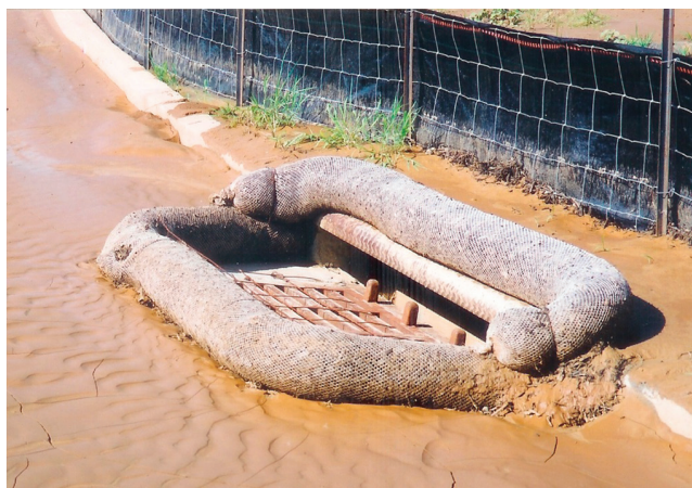
Figure 4 Compost filter sock curb inlet
