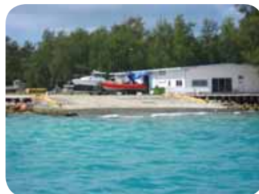
Historic seaplane ramp and existing boathouse
