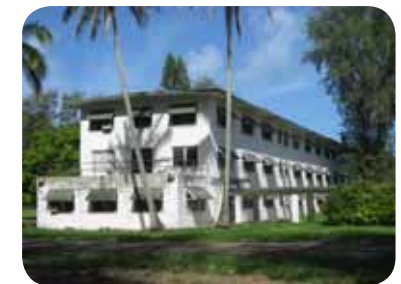
BEQ Barracks: replace with "green-designed" multi-plex units
