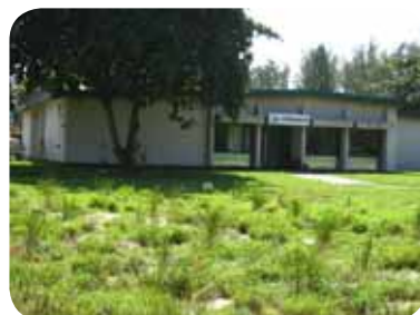
Chugach offices and Medical Clinic
