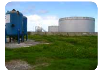
Old fuel tanks located in "no-dig" area
