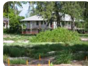
Cable Station building complex
