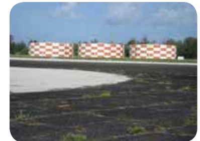
Water collection tanks
