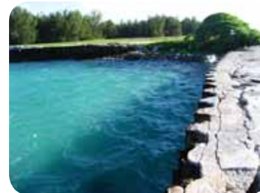
Inner Harbor seawall
