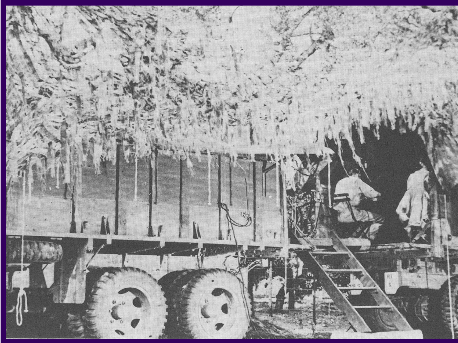
849th SIS Mediterranean Theater (128th SRI), 2 1/2-ton camouflaged intercept van (Photograph from the NSA History Collection)
