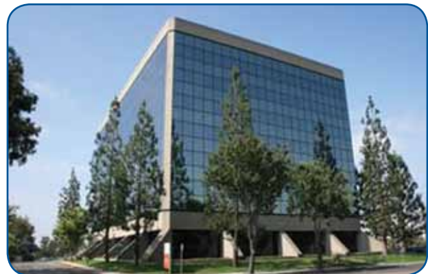
Pictured here is the future site of the OCRCFL.
