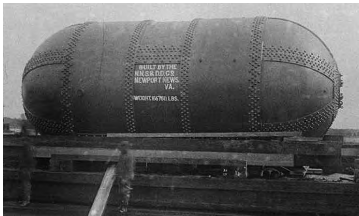
Figure 6. The tank barge docks at Langley.
