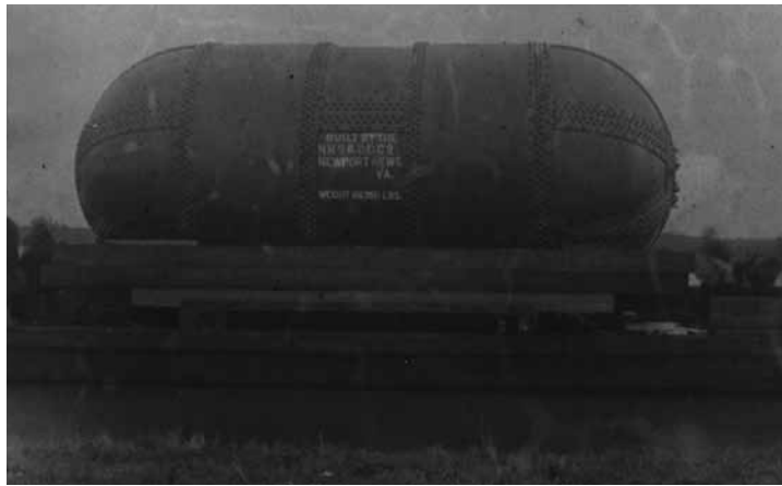
Figure 5. Arrival of the pressure tank of the VDT at Langley via barge in June 1922.
