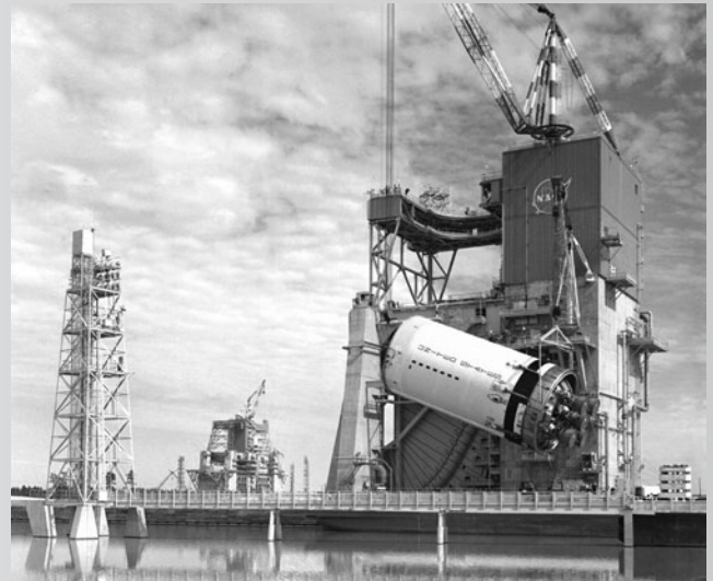
The S-II stage of the Saturn V rocket is hoisted onto the A-2 test stand in 1967 at the Mississippi Test Facility, now Stennis Space Center. This was the second stage of the 364-foot-tall Moon rocket. (NASA image 67-701-C)
