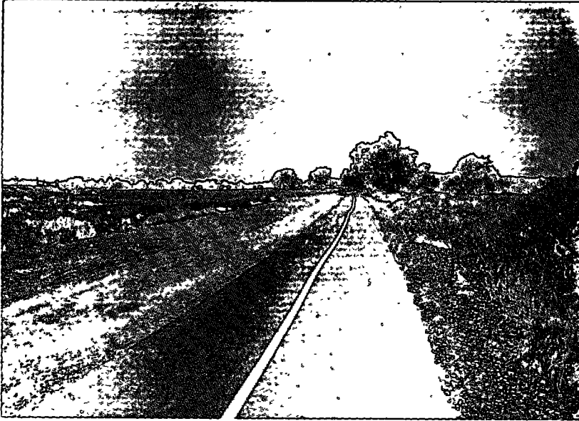
Photo 13. Bikeway at the east end of Rossmoor Bar.
