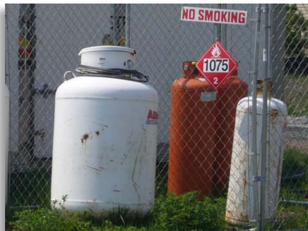
The product inside these liquefied petroleum gas (LPG) containers has a vapor pressure ( V_p ) and vapor density ( V_d ) greater than air.
