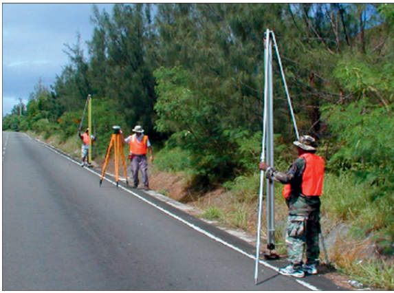
Figure 4. Differential leveling, Commonwealth of the Northern Mariana Islands.
