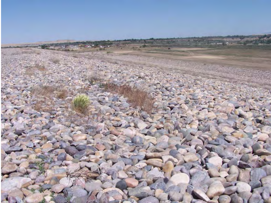
SHP 5/08. PL-1. Depressions in cell side slope rock cover that contain vegetation.
