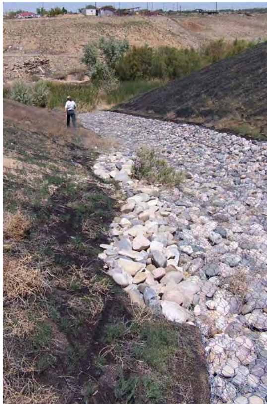
SHP 5/08. PL-2. Repaired area of outflow channel.
