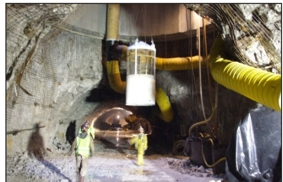
Deep tunnel extension.
