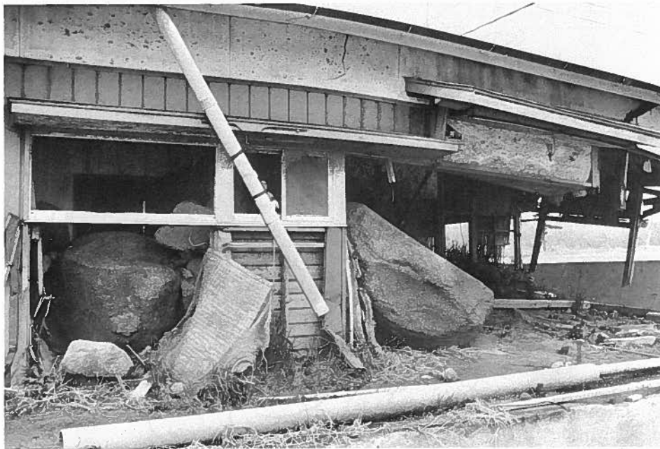
Unzen volcano, Japan. House destroyed and partially buried by lahars in the Mizunashi River valley. Large rounded boulders are blocks of the new lava dome originally deposited by pyroclastic flows in the headwaters of the Mizunashi River and later remobilized by lahars. In this area, the threat of lahars during rainstorms caused thousands of people to evacuate their homes on many occasions. Photograph by S. R. Brantley.
