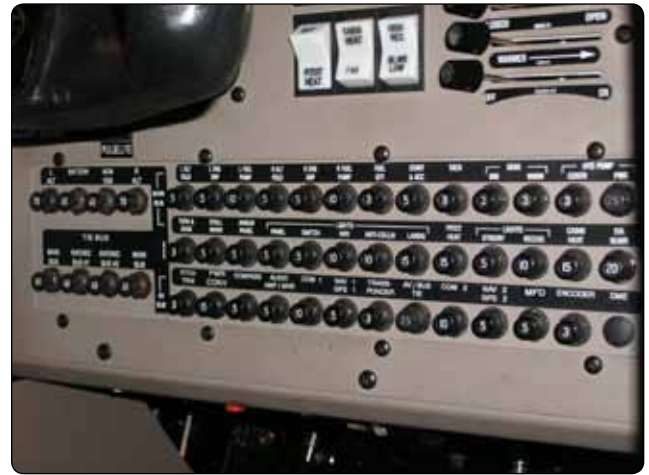
Figure 9-83. Light aircraft circuit breaker panel.
