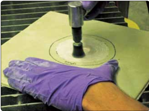
Figure 7-58. Taper sanding of repair area.
