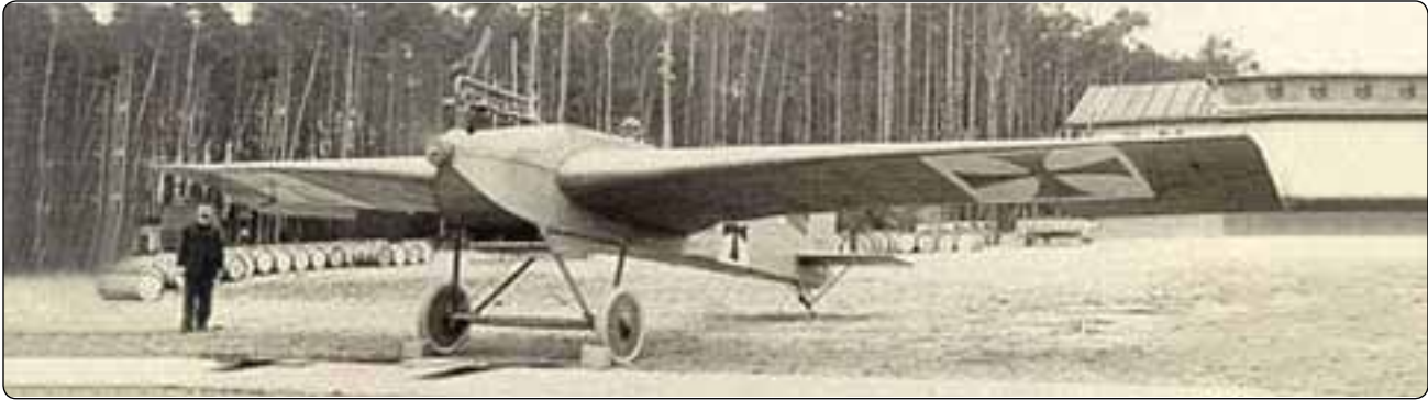
Figure 1-6. The Junker J-1 all metal construction in 1910.
