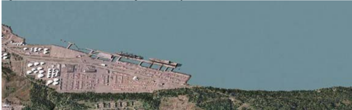
Figure 3. Port in 2005; Prior to Expansion Project Activities. Source: ICRC, 2010.
