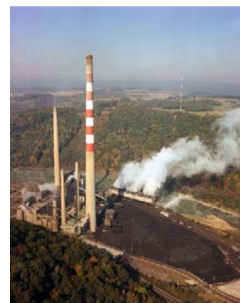
Photo Courtesy of NREL. Shawville Station biomass cofiring plant.
