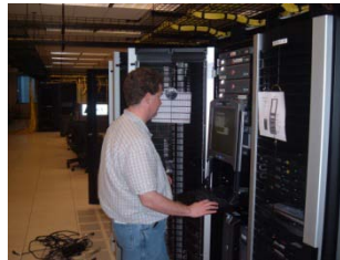
Work continues throughout the night.
