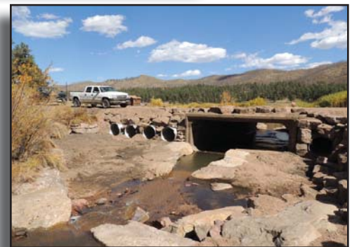
Culvert passing through where Trail and West Creek merge. Flood stage culvert was implemented to connect floodplain at high stage flows.
