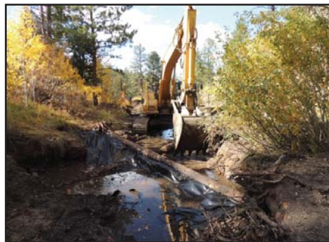
Construction of wood structures on steeper reach of Trail Creek
