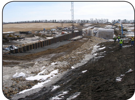
Devil’s Lake – Tolna Outlet - Construction March 2012
