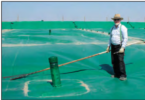
A MT producer captures the methane as part of their manure management plan.
