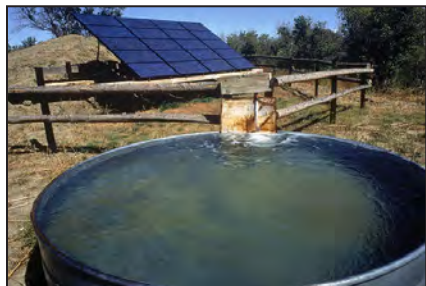
Solar panels provide energy to pump water to livestock.
