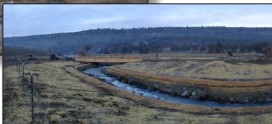
A constructed fish passage in OR goes around a dam to allow various species to swim upstream and spawn.
