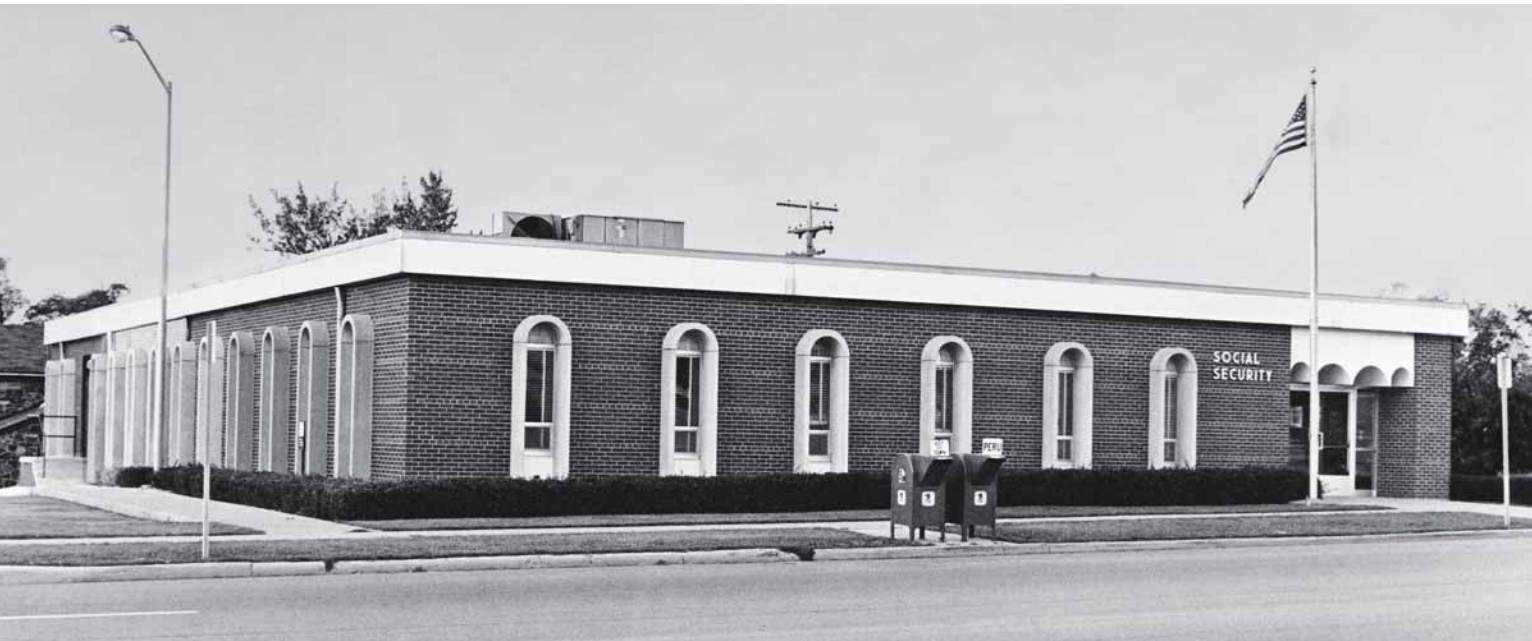
SOCIAL SECURITY ADMINISTRATION DISTRICT OFFICE BUILDING, PERU, ILLINOIS OMARA & CHAMLIN | 1969
