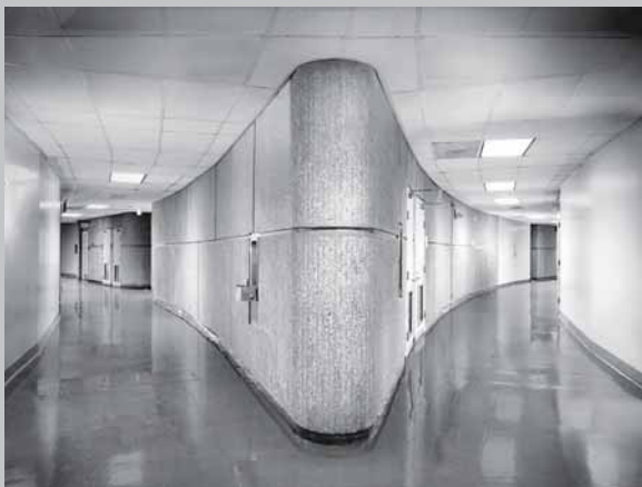
ROBERT C. WEAVER FEDERAL BUILDING, U.S. DEPARTMENT OF HOUSING AND URBAN DEVELOPMENT HEADQUARTERS, WASHINGTON, DC | MARCEL BREUER | 1963-68 ABOVE: TYPICAL INTERIOR CORRIDOR
