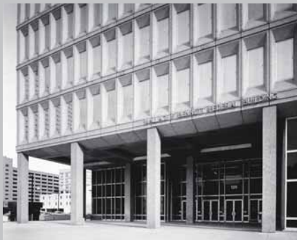
ENTRANCE SHOWN BEFORE UPGRADES (ABOVE), AND AFTER UPGRADES HAD BEEN COMPLETED (UPPER RIGHT).
