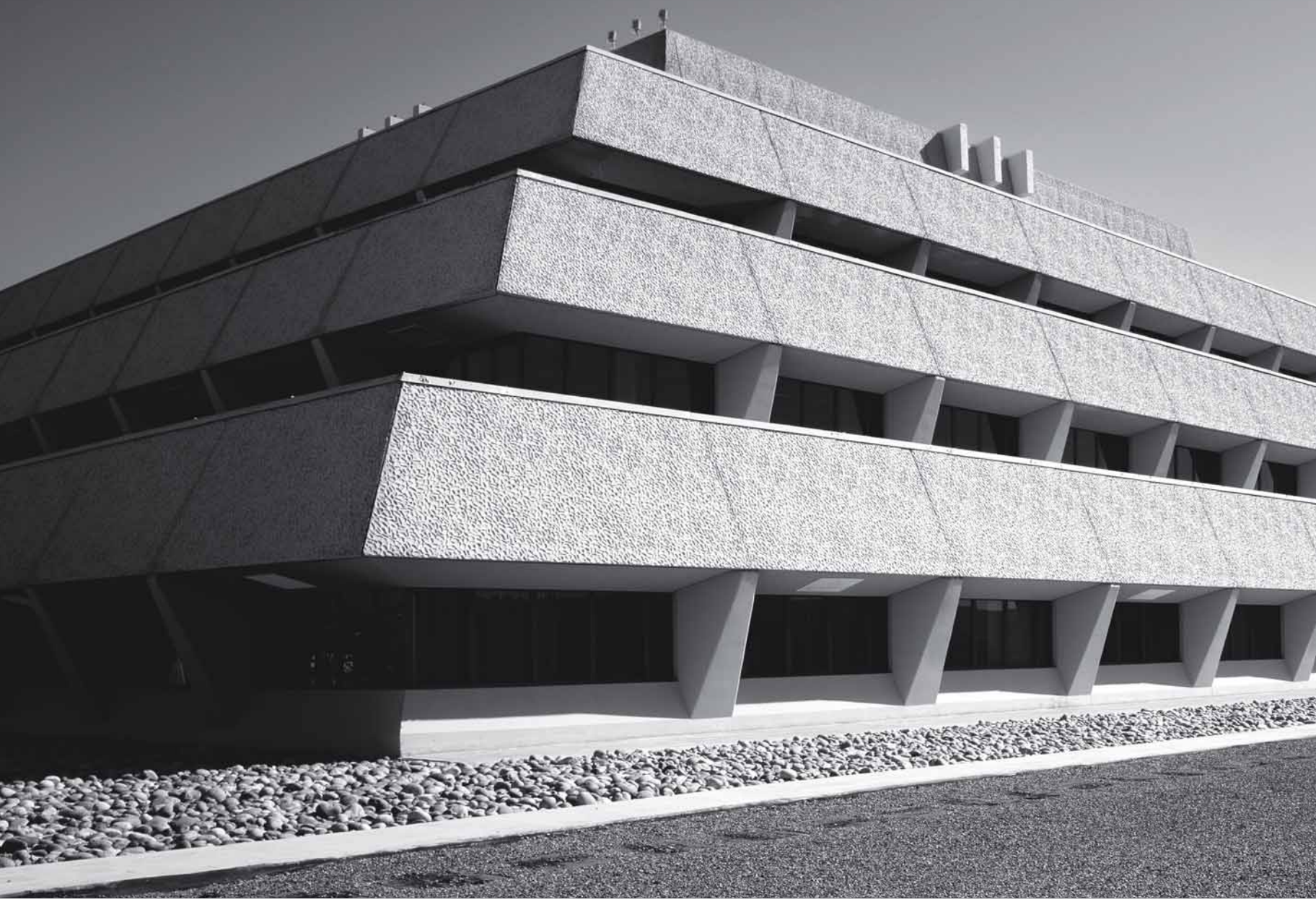
CHET HOLIFIELD FEDERAL BUILDING, LAGUNA NIGUEL, CALIFORNIA | WILLIAM L. PEREIRA & ASSOCIATES | 1971 | ACQUIRED BY GSA IN 1974
