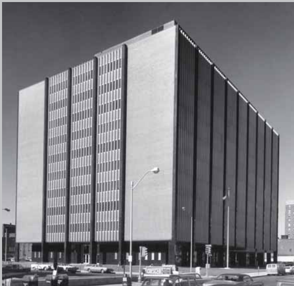
NORTHWEST VIEW SHOWN BEFORE FACADE REPLACEMENT (ABOVE) AND AFTER (RIGHT).
