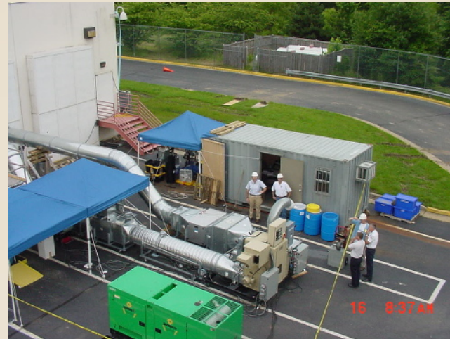
VHP fumigation at Dept of State
