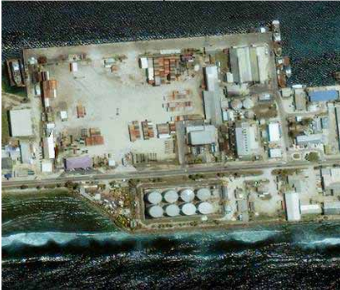
MEC Fuel Storage and Power Plant on Majuro
