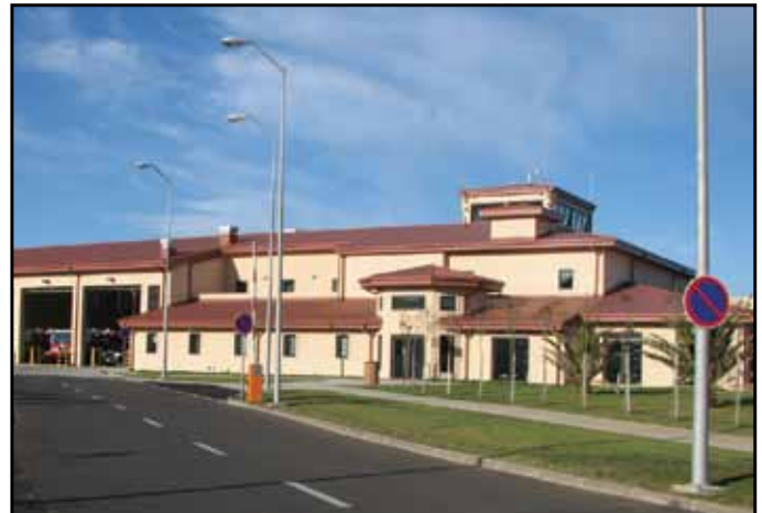
The Lajes Field fire department at its new facility, 2011. (Courtesy photo)
