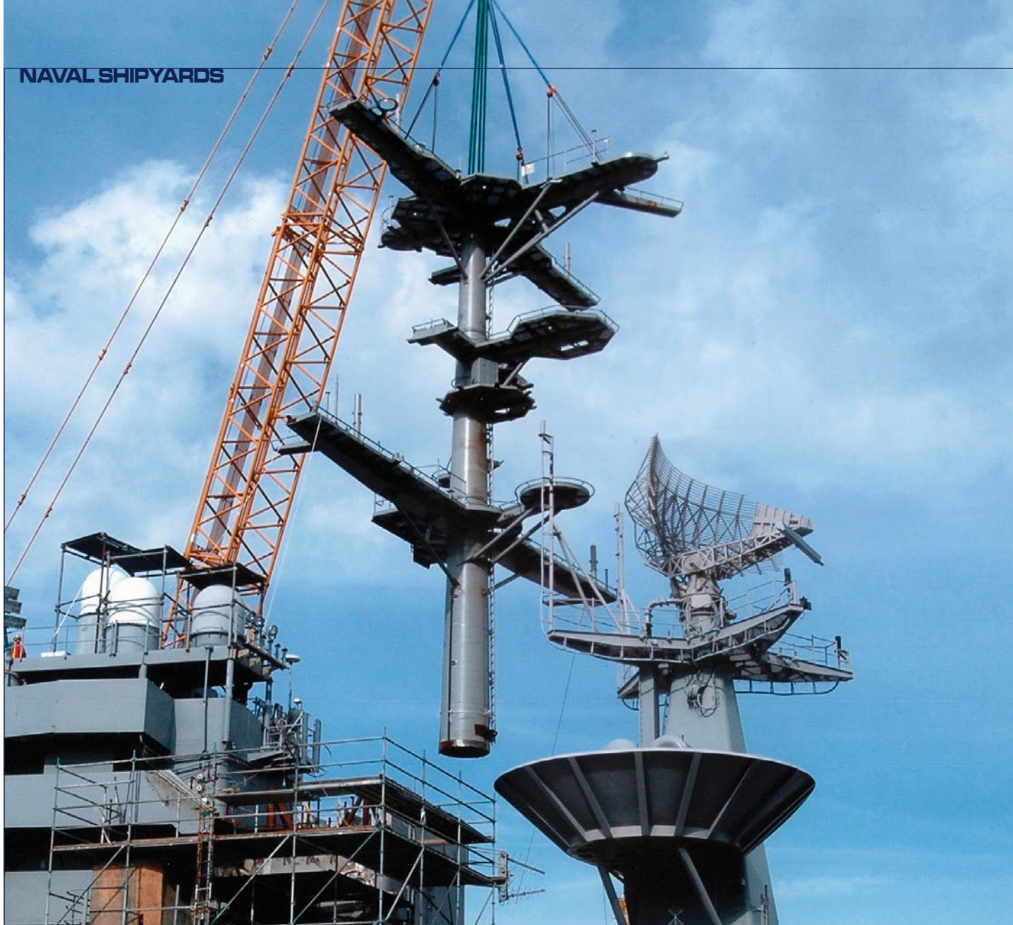
Top During its nearly year-long Planned Incremental Availability plus Docking at Norfolk Naval Shipyard, USS George Washington (CVN 73) had a collection of ship alterations performed, including major upgrades to the combat systems suite, known as Capstone. A highlight of the Capstone process was the installation of a new carrier mast strong enough to support the combat system upgrades in January 2007. Thanks to extensive prefabrication work performed pier-side, a significant time-saver for the project team was having the new mast installed in a single lift, when previous installations required three separate lifts. Bottom A second generation Portsmouth Naval Shipyard employee, Plastic Fabricator Apprentice Steven Bachmann, and his father, Plastic Fabricator Mechanic Kenneth Bachmann, oversee the Teflon coating process applied to ship ball valves.
