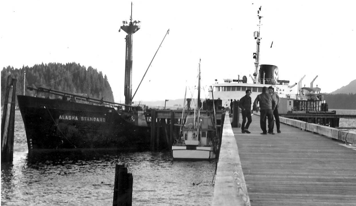
Fig. 4. The Alaska Standard docked at Ouzinkie, Alaska, ca. 1967, after the dock was rebuilt following the 1964 earthquake. Photograph by Timothy Smith, Fontana, California, used by permission.
