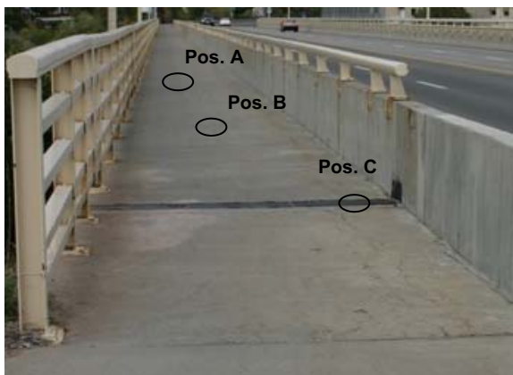
Figure 3: Temperature measurement locations along the Omega Bridge.
