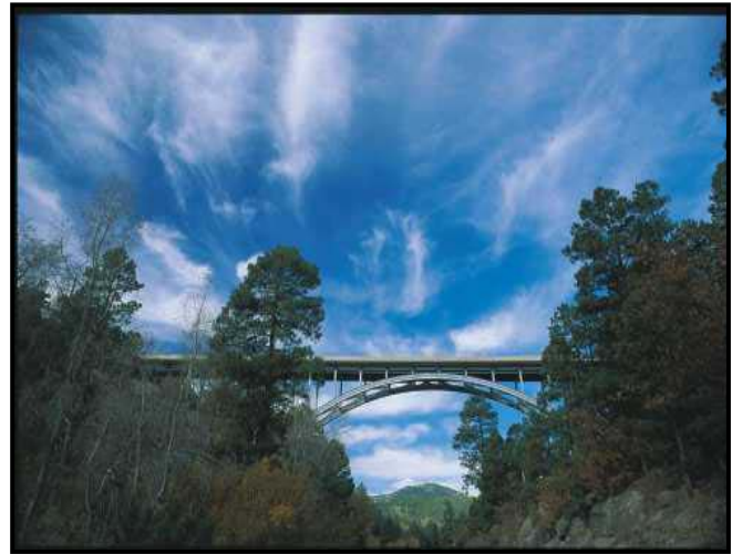
Figure 1: Vibration and temperature measurements were taken along the Omega bridge in Los Alamos, NM in July 2008.
