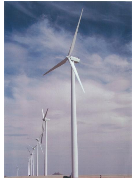
Fig. 2: 1.5MW GE wind turbines at the Colorado Green & Twin Buttes Wind power project.
