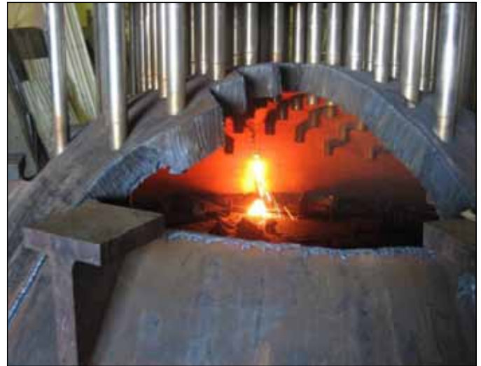
Figure 9.14 Sectioning of reactor vessel head penetrations from WNP-1, a cancelled plant
