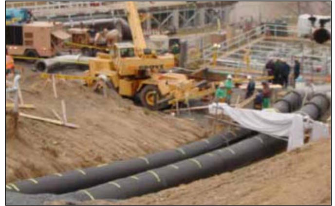
Figure 9.27 Installation of underground Class 3 safety-related HDPE piping
