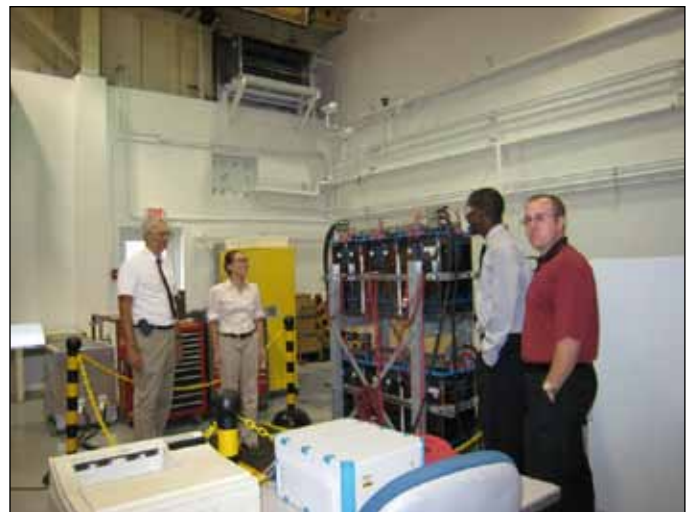
Figure 10.5 NRC staff reviewing the first set of batteries that the contractor has received before commencing confirmatory battery testing
