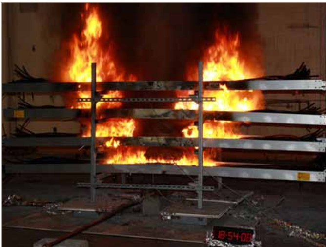
Figure 7.10 Burning cables during cable tray fire test (Side view of burning cables in trays during a multi-tray test after ignition using a small gas burner)
