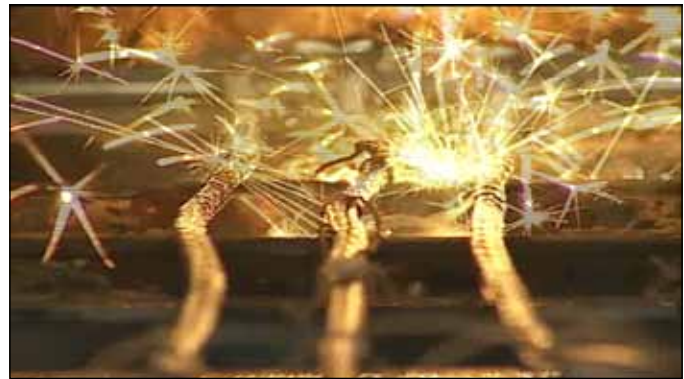
Figure 7.12 Direct current electrical cable hot short
