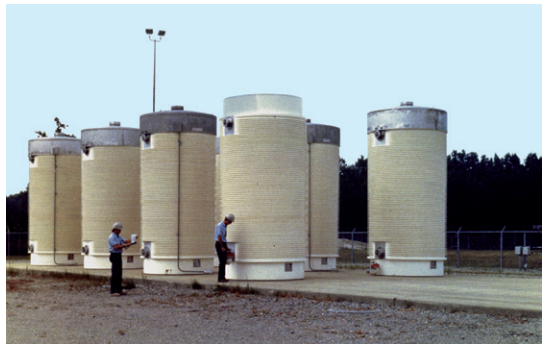
Independent spent fuel storage installations are used to safely store spent fuel.
