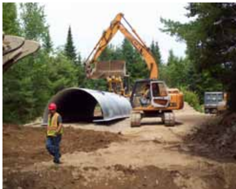
Salmon Habitat and River Restoration Project, culvert replacement. (Credit: NOAA)
