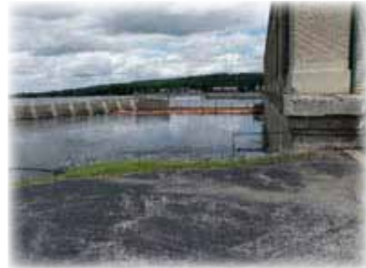
Army Corps of Engineers dam and lock at Green Island near Troy, New York Credit: Stephen Patch/USFWS
