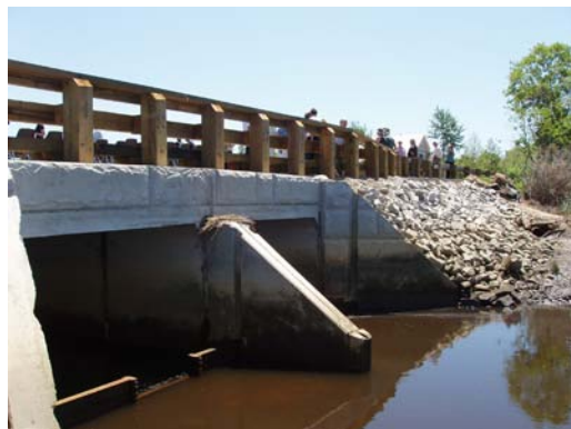
Newly installed culverts. Photo credit: NOAA
