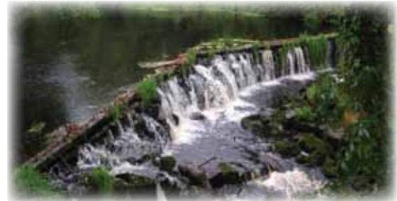
The Rhode Island River Ecosystem Restoration will remove the Lower Shannock Dam (above) on the upper Pawcatuck River. Credit: NOAA
