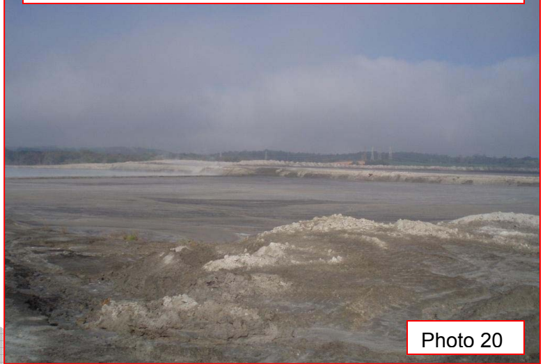
Gypsum Stack -southeast side - looking west
