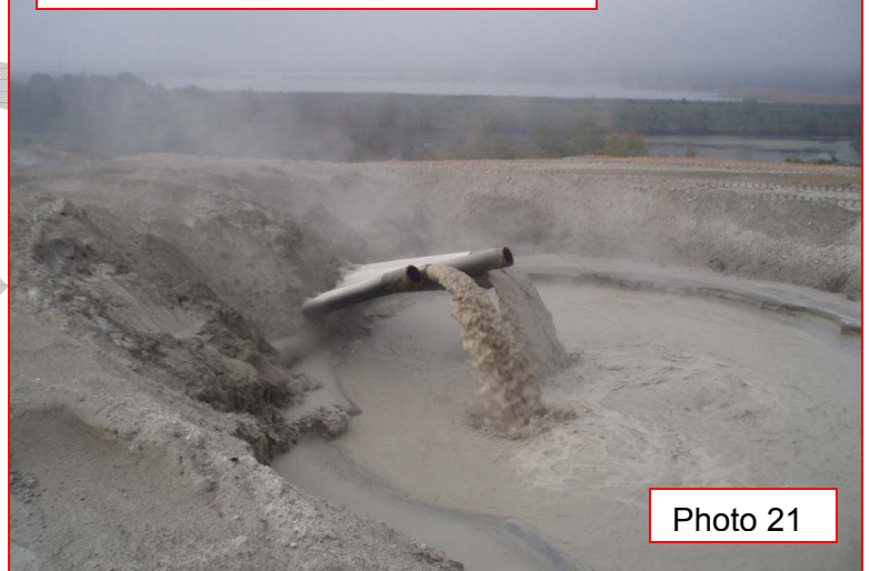
Slurry Pipes near northwest corner
