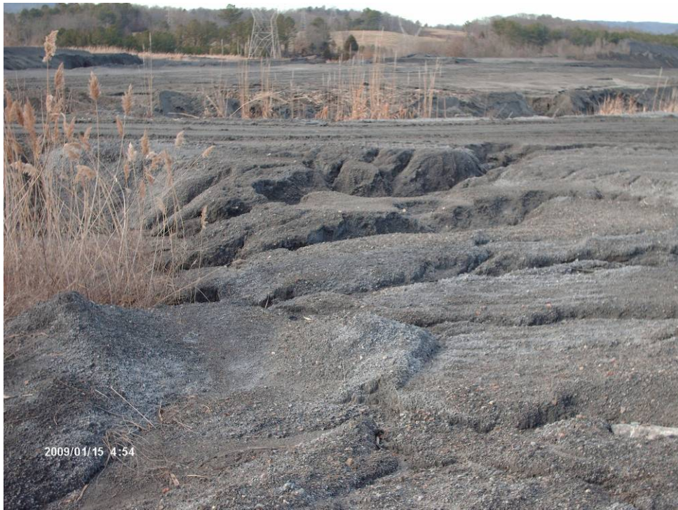
Figure 14. Typical Roadway/Surface Rills, 2009
