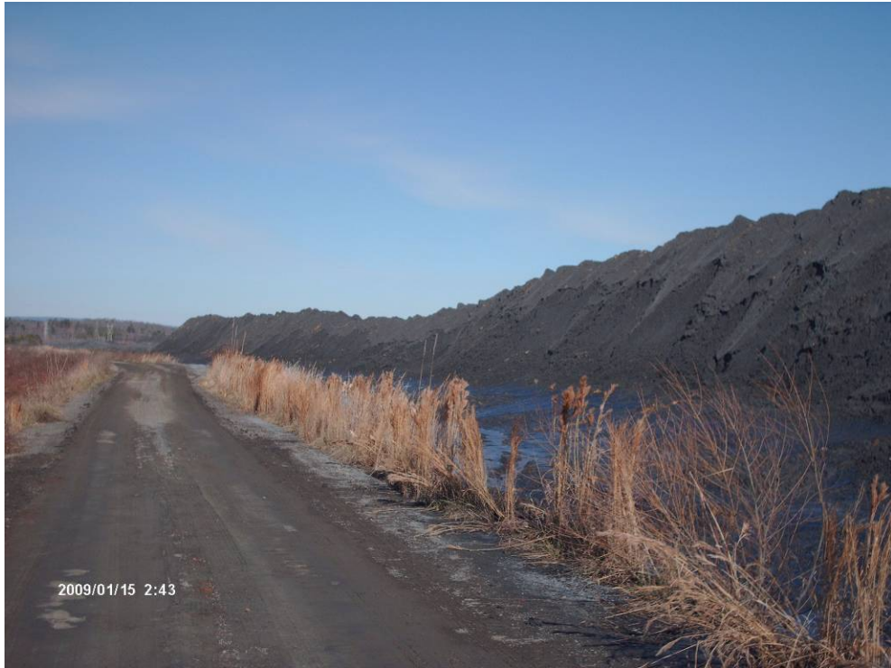
Figure 13. Typical Surface Ditch, 2009
