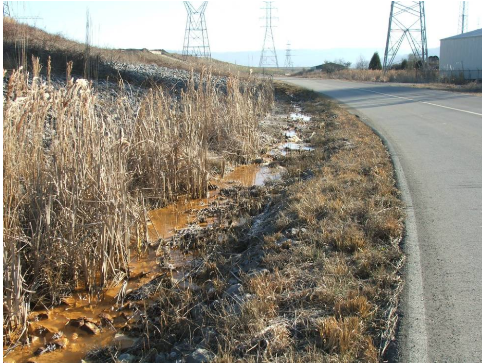
Figure 18. Ditch/Seepage Conditions along Scrubber Road, 2009
