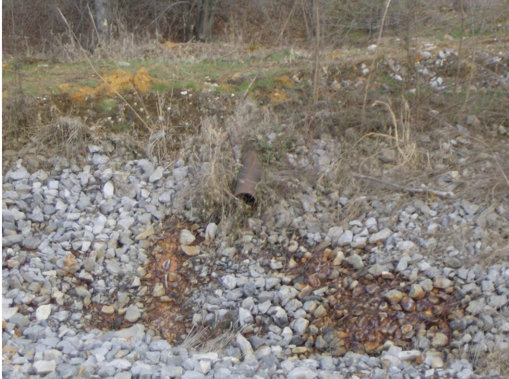
Figure 20. Discharge Pipe along Scrubber Road, 2009
