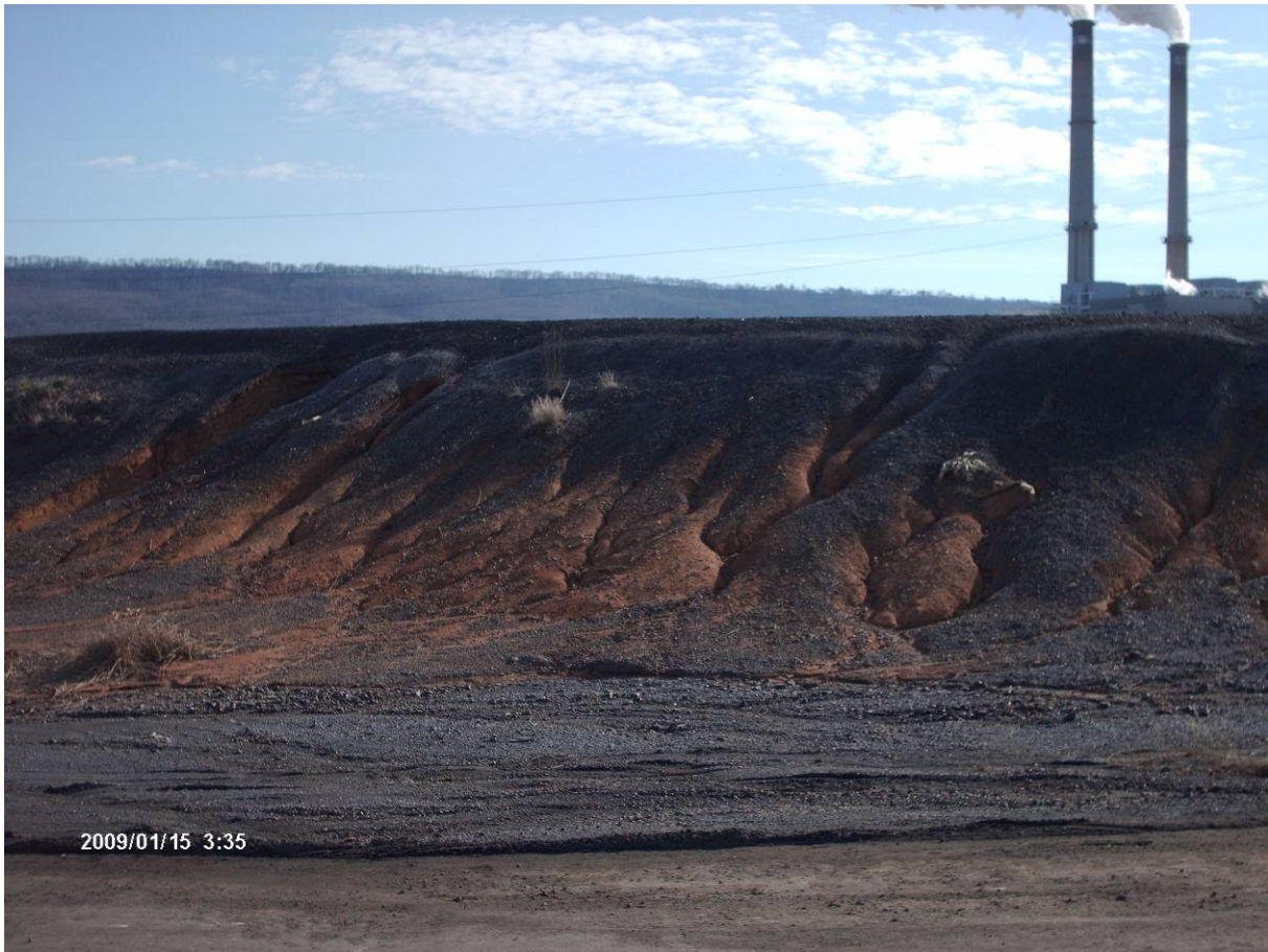
Figure 12. Typical Rill Erosion, 2009
