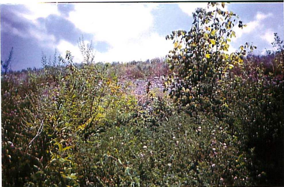
View of dike slope showing previous repair protected with using riprap.
