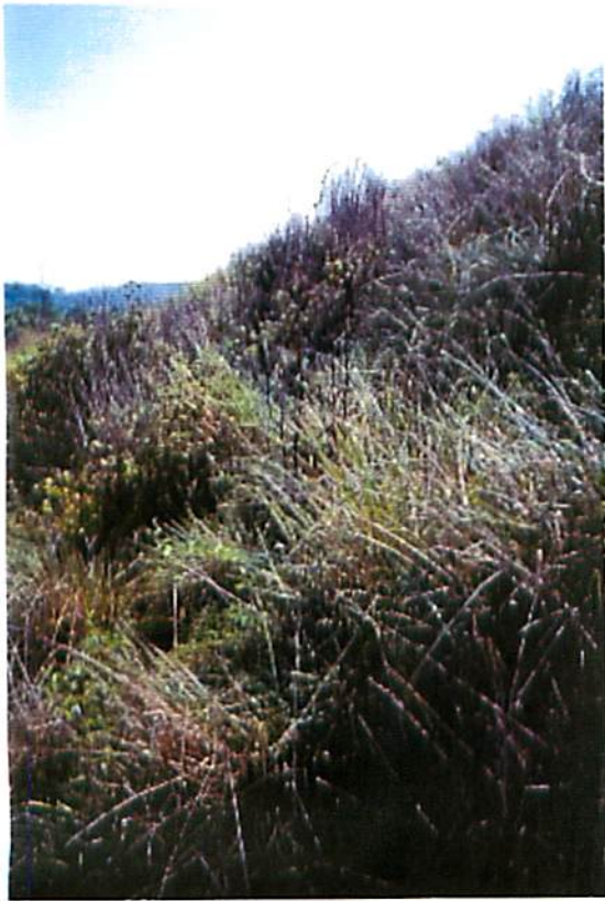
View of dike's downstream slope
