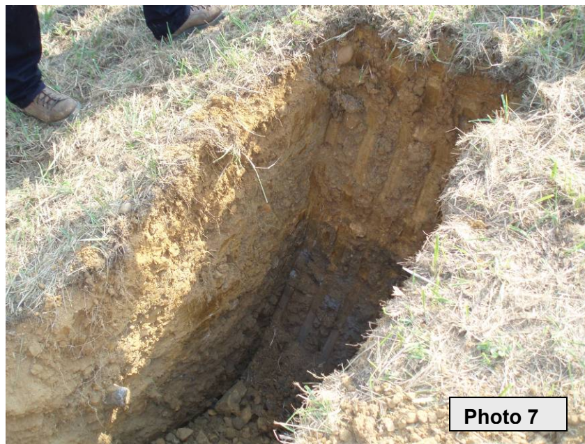
Photo 7. North Side of Dry Stack. Slough in 2007.
