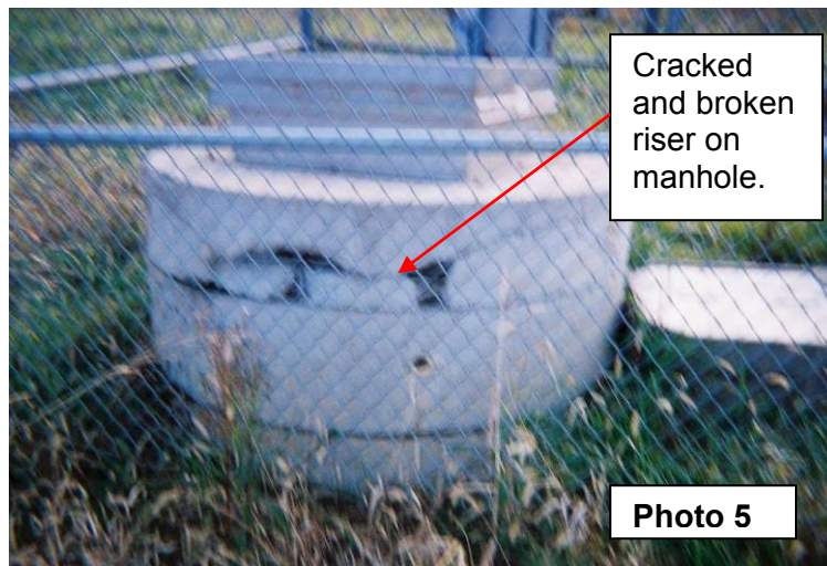
Photo 5. Northeast Seepage Collection Manhole.
