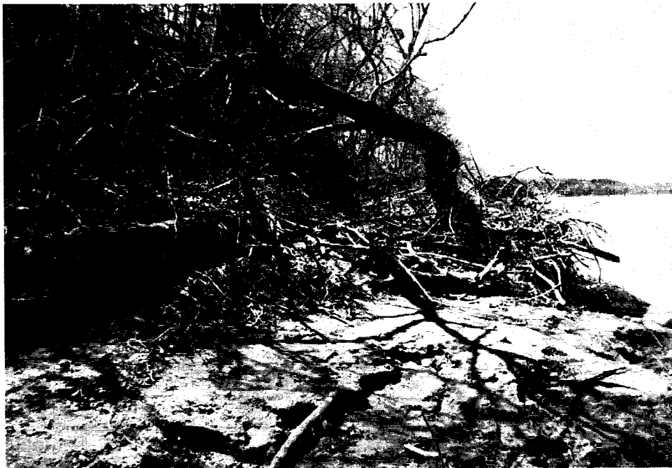
PICTURE 6 - TREES ALONG THE TOE OF DIKE UPROOTED AND FALLEN INTO CHEROKEE RESERVOIR
