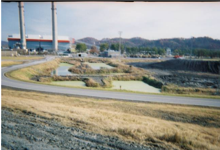
Photo 16. Coal Yard Drainage Basin.
