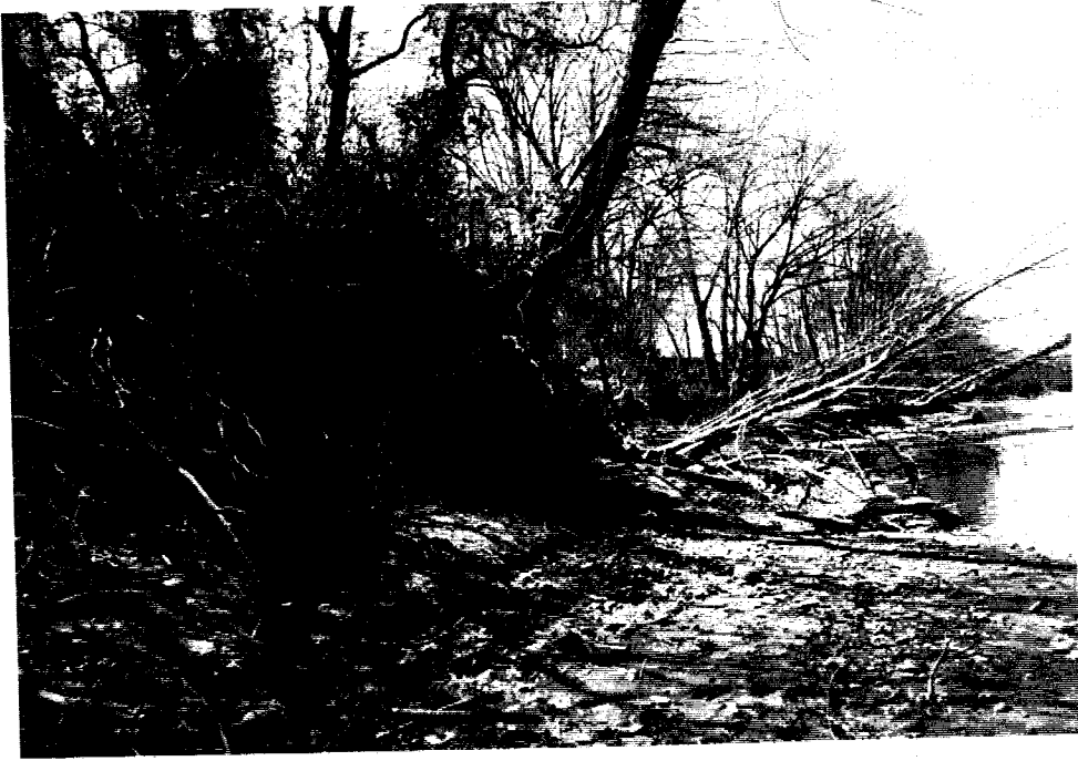
PICTURE 5 - TREES ALONG THE TOE OF DIKE THAT HAVE UPROOTED
