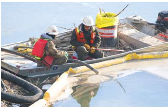
Cenospheres are collected through a hose connected to a vacuum truck.
