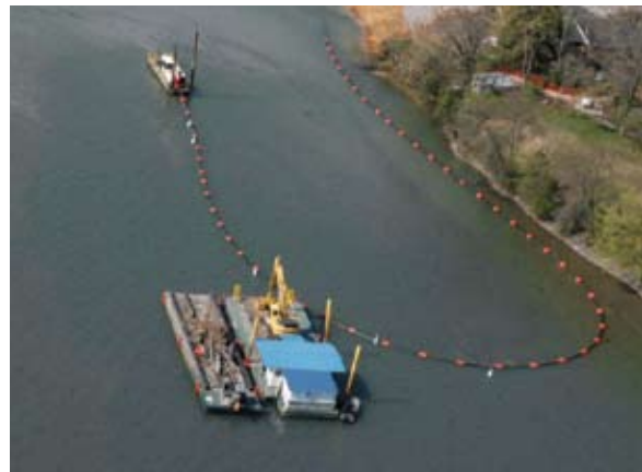
Dredges have removed more than 156,000 cubic yards of ash from the main channel of the Emory River.
