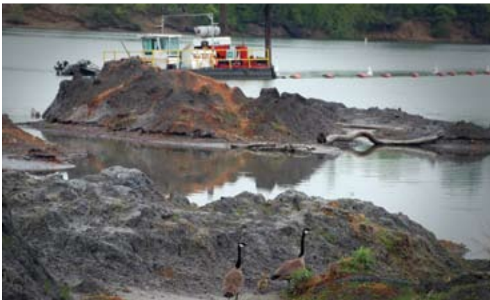
Dredges have removed more than 156,000 cubic yards of ash from the main channel of the Emory River.
