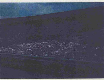
Based on the site reconnaissance, piping and excessive seepage was hypothesized to be the triggering mechanisms for the "blow-out".
