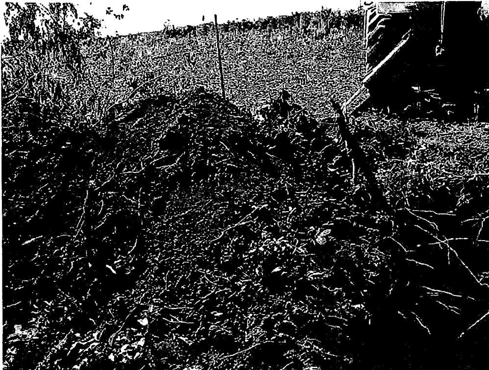
Photograph 10 - Materials excavated from Observation Trench OT-5.
