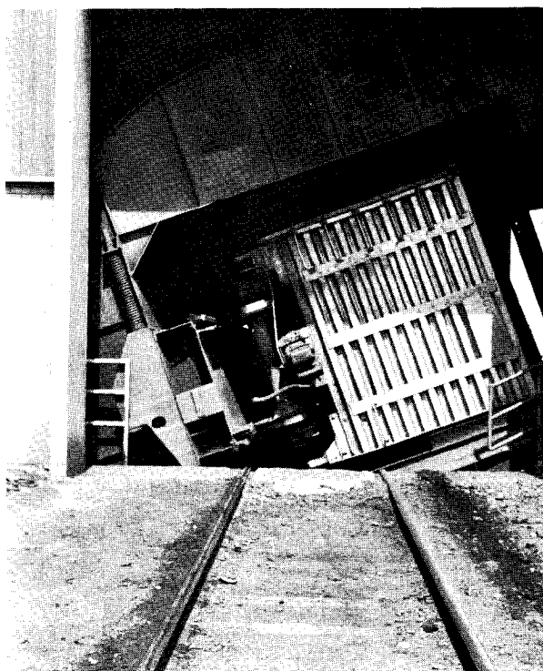
FIGURE 61.—Each of two car dumpers has a capacity of twenty 50-ton cars per hour.
