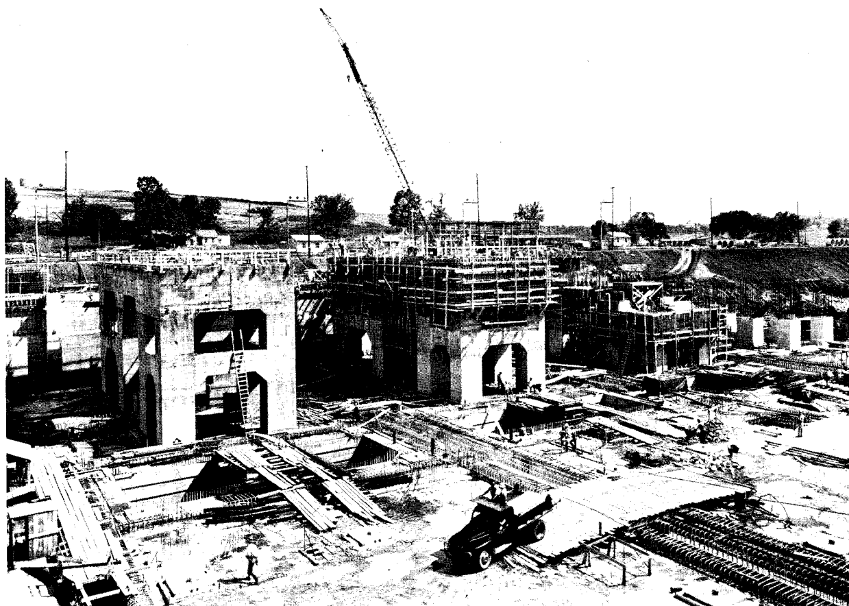
FIGURE 95.—Construction progress as of August 19, 1952, showing turbogenerator foundations in progressive stages of construction, units 1-4 reading left to right.
