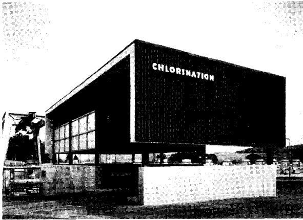
FIGURE 51.—Chlorination building. Intermittent doses of chlorine, through diffusers located beneath the intakes of the condenser circulating water pumps, inhibit slime growth in water passages and condenser tubes.
