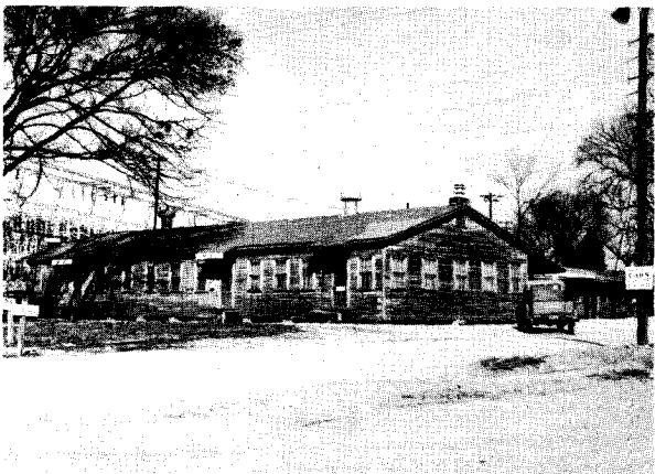
FIGURE 83.—Personnel and time office building. Eight clock alleys at the rear passed 2080 men on day shift in five minutes.
