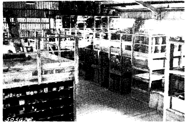
FIGURE 88.—The main warehouse building, of structural steel construction, was divided one-fifth for office space, one-fifth for construction material, and the remaining space for permanent material. Erection of steel and wooden bins allowed maximum utilization of available space.
