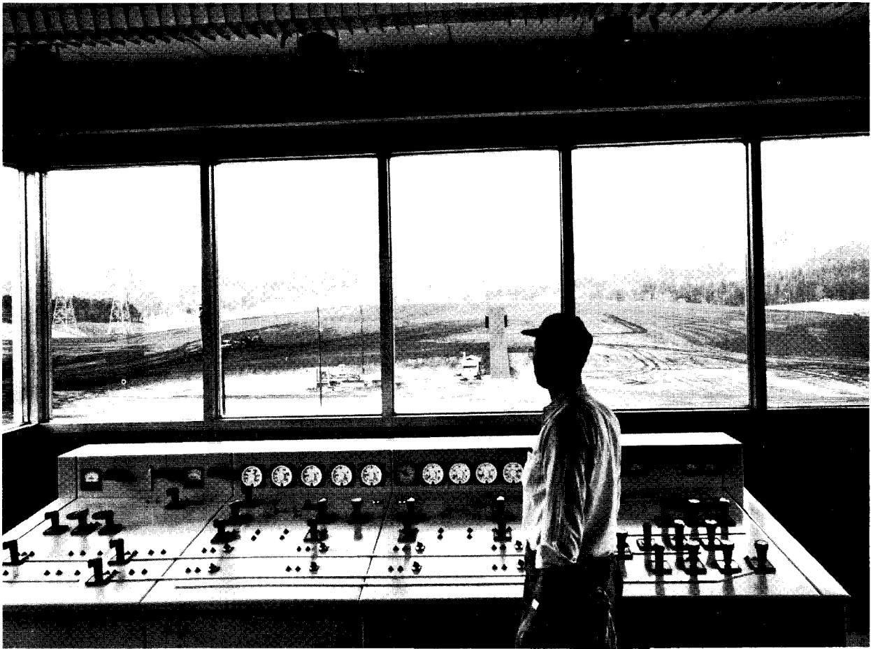
FIGURE 65.—The control room for the coal handling system, glass enclosed on three sides, is located on top of the conveyor control building and provides an unobstructed view of the entire operation.
