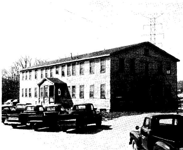
FIGURE 82.—The administration building was a 2-story unpainted structure. A 2-story brick vault at the rear provided fire-proof storage for engineering and accounting records.
