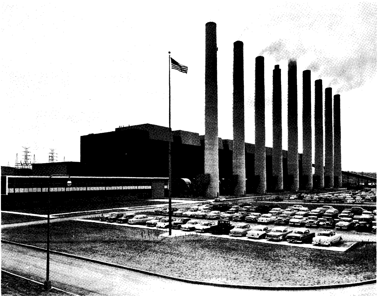
FIGURE 11.—Kingston powerhouse looking south. The dark wall mass of the maroon, steel-paneled boiler bay contrasts with the gray brick and glass exterior of the office wing and the concrete stacks.
