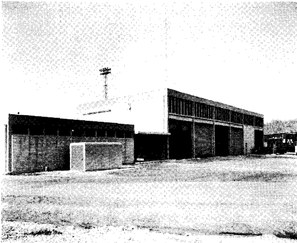
FIGURE 66.—The utility building is centrally located near the crusher building and houses facilities for servicing all mobile equipment used in coal handling operations.
