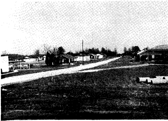
FIGURE 72.—Laddie Village Addition consisting of 20 homes and lots in the suburbs of Kingston was purchased for employee housing.
