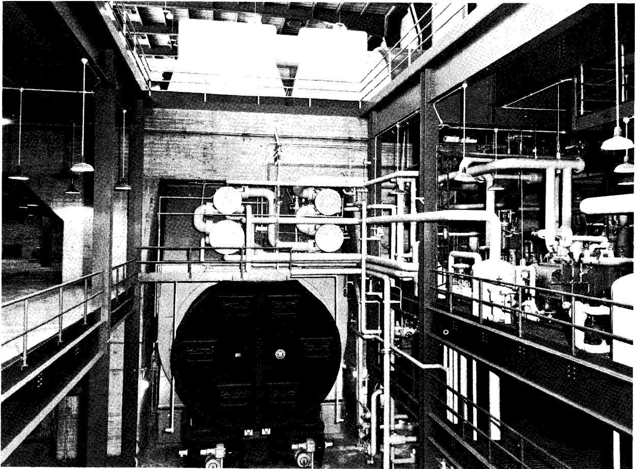
FIGURE 24.—Unit 6 turbogenerator, its low-pressure feedwater heaters and condenser. At right, steam jet air ejector.
