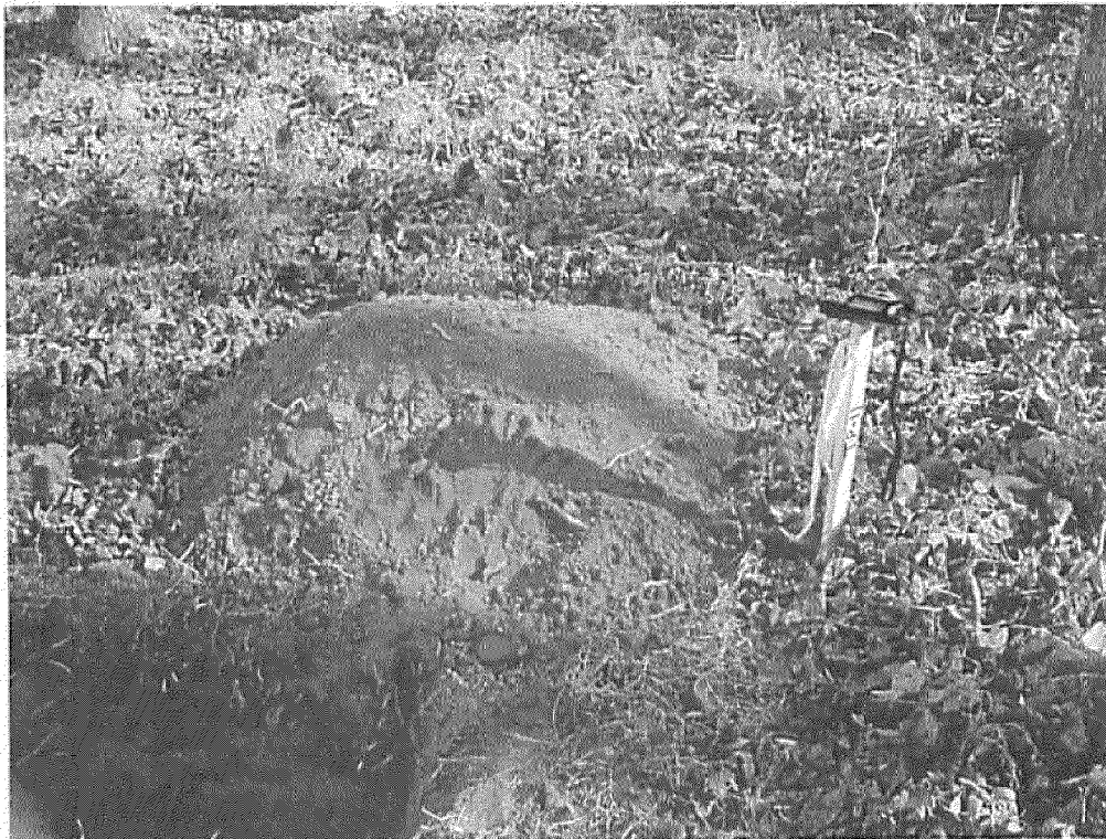
Photograph 22 – Materials excavated from Observation Trench OT-11.
