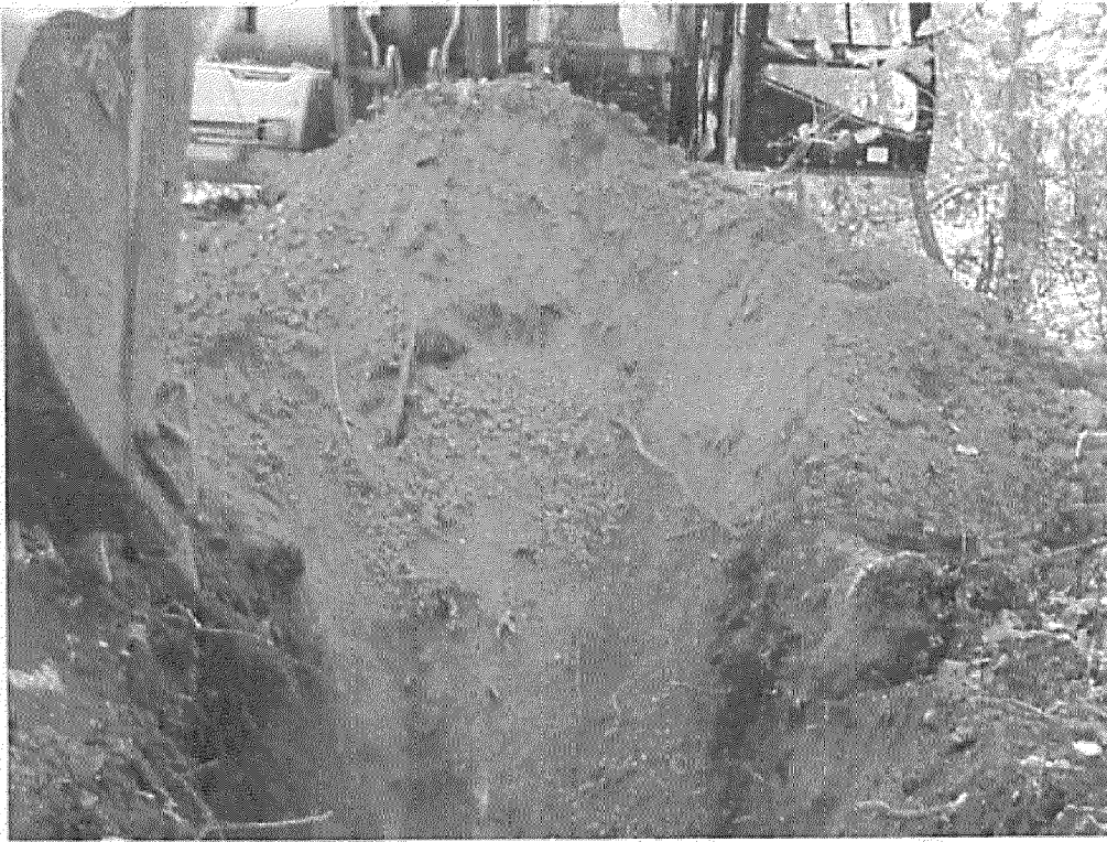
Photograph 4 – Materials excavated from Observation Trench OT-2.
