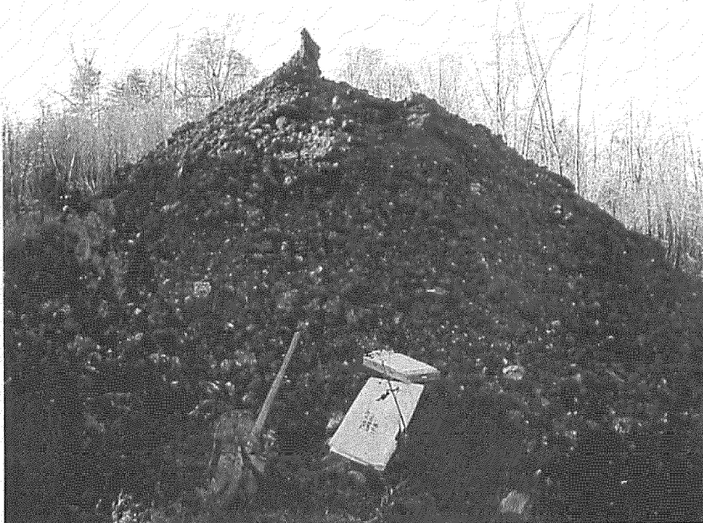
Photograph 16 – Materials excavated from Observation Trench OT-8.
