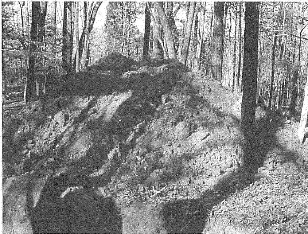
Photograph 12 – Materials excavated from Observation Trench OT-6.
