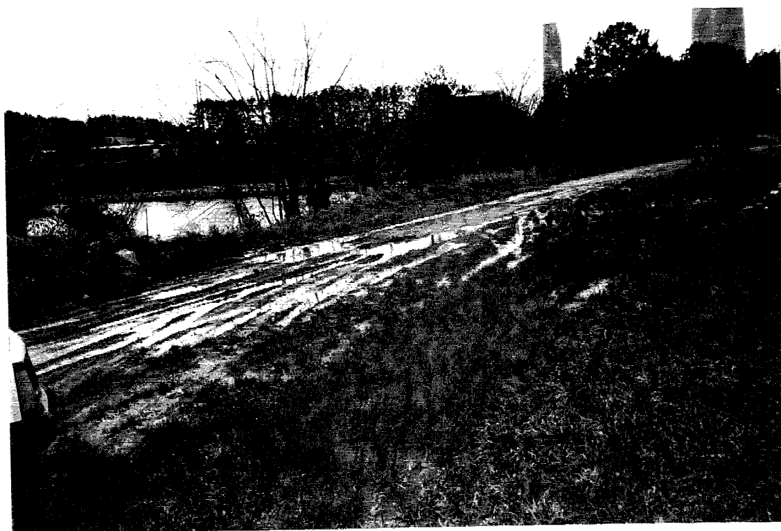
Figure 4. Rutting on access road south of the engineered wetlands due to ALD clog.
