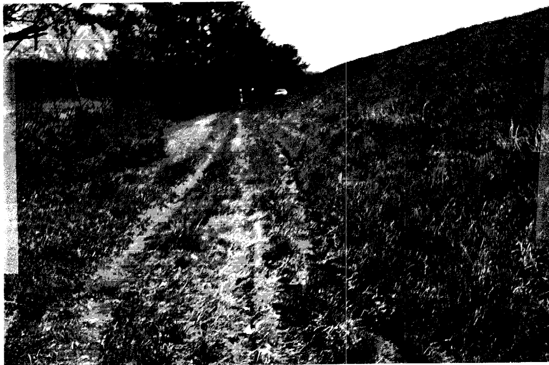
RUTTED AREAS - WEST END OF DIKE "C"
