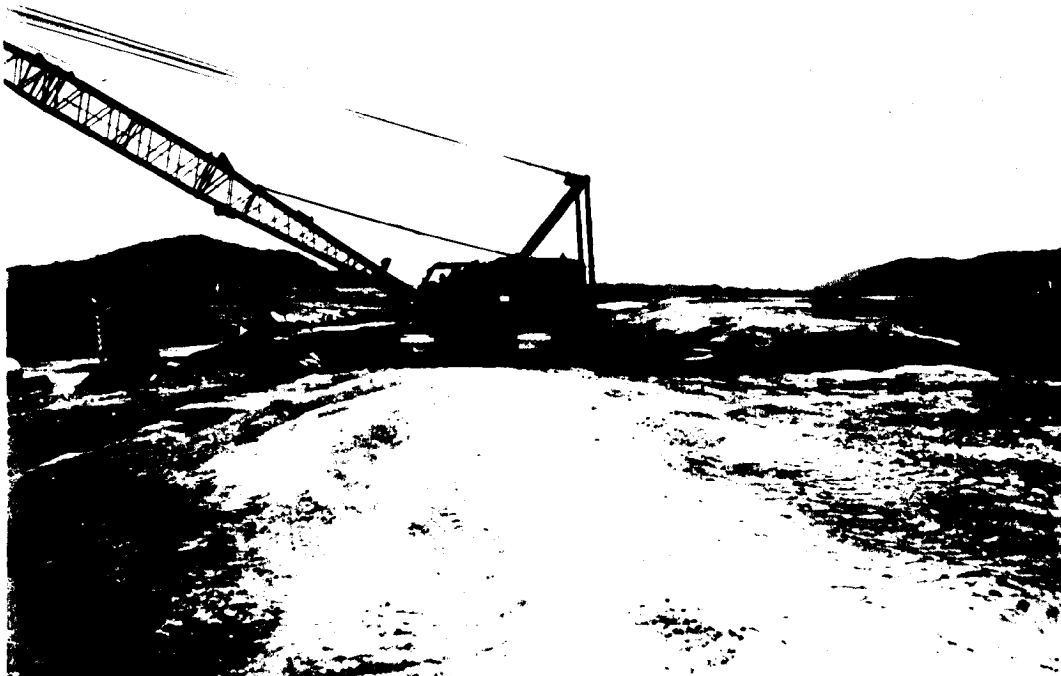
④ RECLAIMING ASH FROM DISCHARGE.
